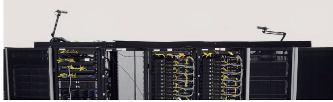
Fig. 3. The prototype of mmWave radios are equipped on the racks in cloud center.
